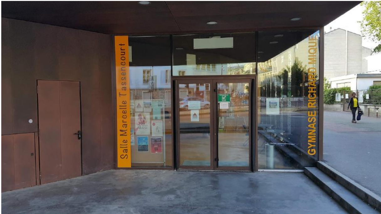
Figure 11: Hall Marcelle Tassencourt /Gymnasium Richard Mique (Yves Richard, 2016)
