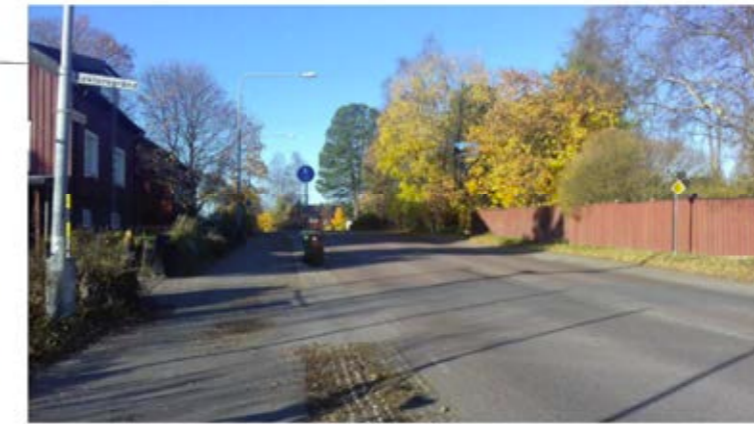
Bölevägen in the autumn, on the right side sidewalks are missing. On the left side there is a substandard bicycle lane. Street development program (Photo: Inger Engström, 2016)
