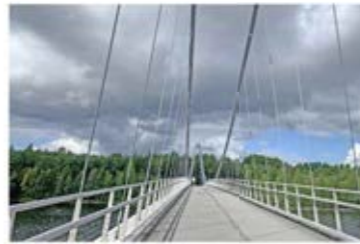
The new bridge, Lundabron. Photo Olov Hjærtström Åaudin 2021
