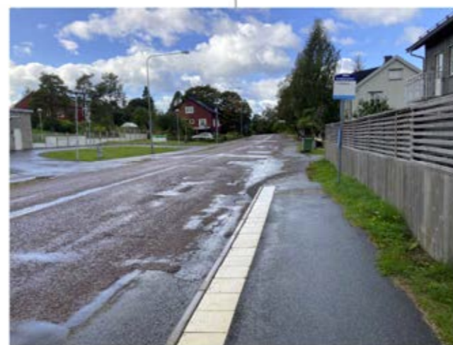
Pictures of Bölevägen and its surroundings. A narrow bus stop where no wheelchairs can board the bus. (Photo: Eva Maaherra Lövheim, 2021).
