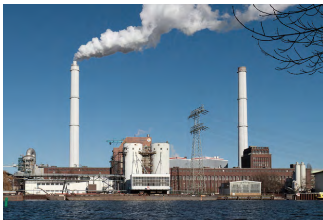
Fig. 19: Power Station Klingenberg in Berlin-Rummelsburg.
