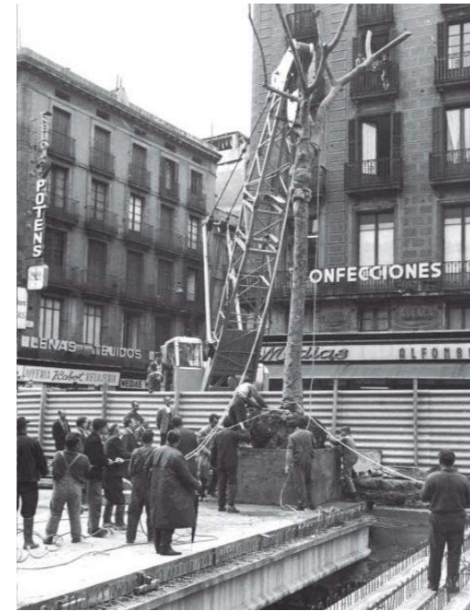
Liceu metro construction work 1968
